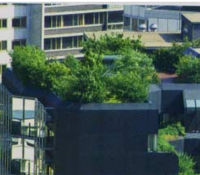
An accessible intensive condominium green roof in Germany
