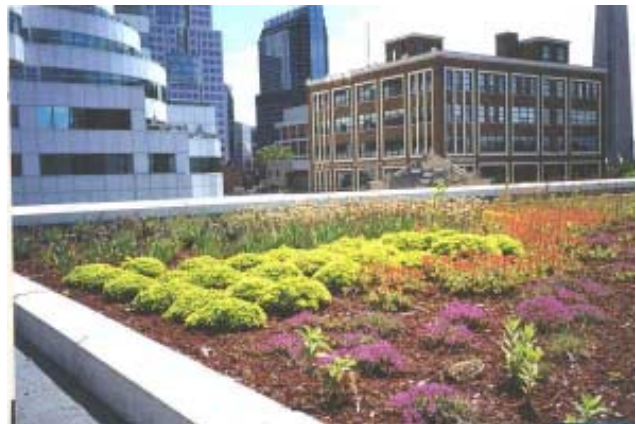
Mountain Equipment Co-op Green Roof, Toronto, Canada
