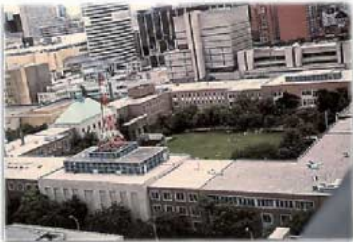
ACCESSIBLE GREEN ROOF, RYERSON POLYTECHNICAL UNIVERSITY, TORONTO, ONTARIO
