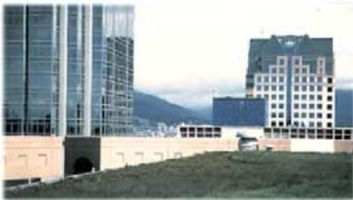
GREEN ROOF, VANCOUVER PUBLIC LIBRARY, BRITISH COLUMBIA
