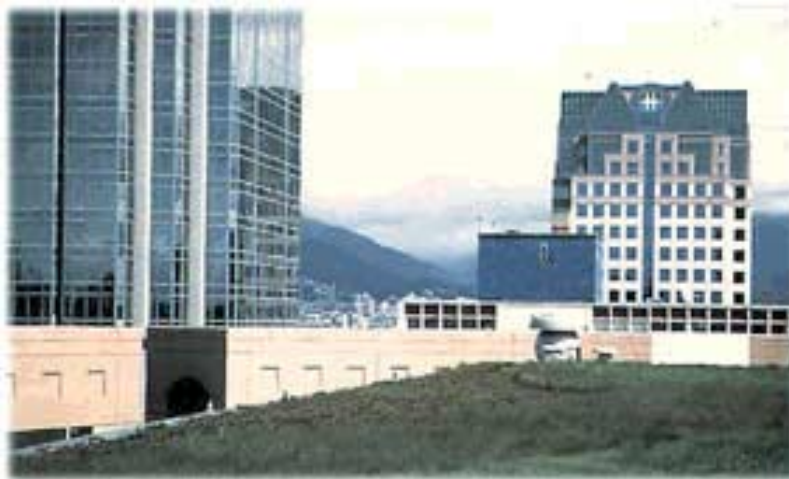
Green Roof, Vancouver Public Library, British Columbia
