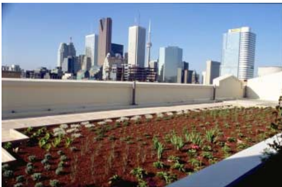
EXTENSIVE GREEN ROOF ON NEW MERCHANDISE LOFTS, TORONTO, ONTARIO
